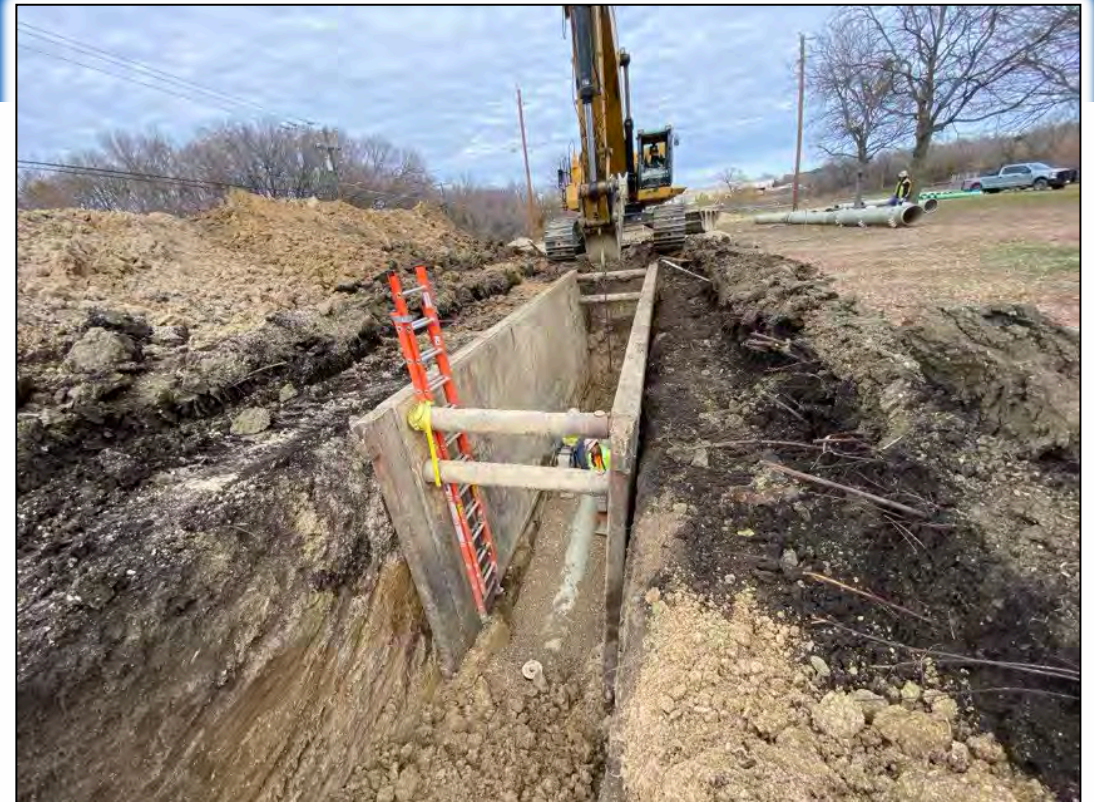
(Example Open Cut/Trenching Pipe Installation)
